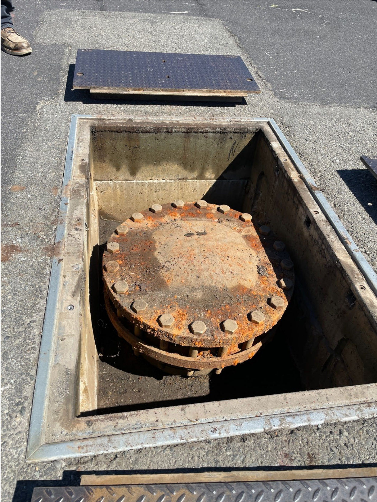
North bypass vault from underground portion
