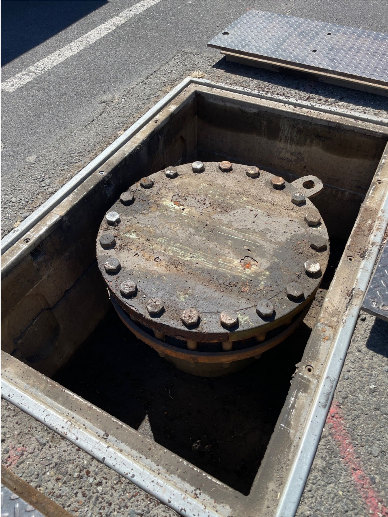
South bypass vault to underground portion
