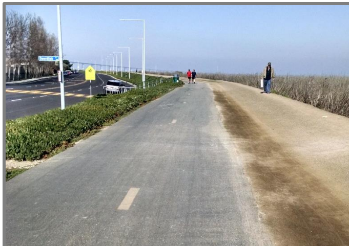
Figure 6-2. Foster City Levee Section with Adjacent Levee Crest Higher than Pedway
