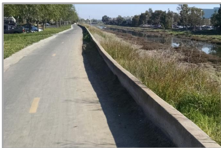
Figure 6-5. Floodwall along Belmont Slough
