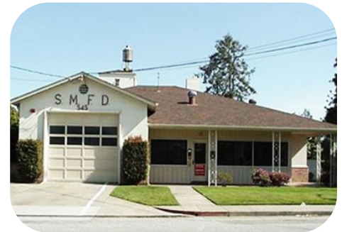
San Mateo Station 25—545 Barneson Ave. Engine 25—3 personnel
