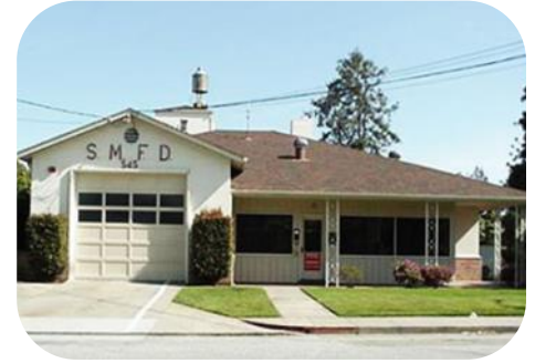
San Mateo Station 25—545 Barneson Ave. Engine 25—3 personnel
