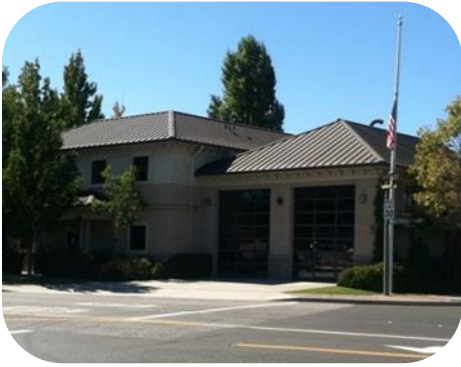
Belmont Station 14—911 Granada St. Engine 14—3 personnel Hazmat 14—cross staffed
