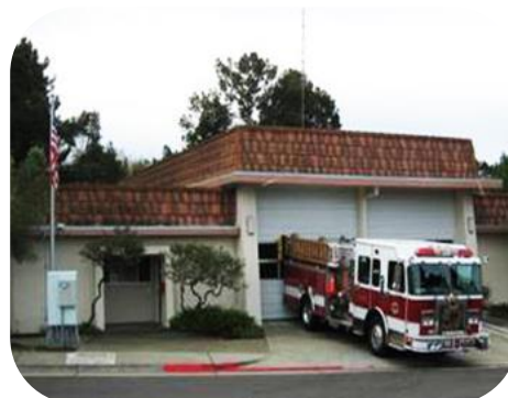
San Mateo Station 27—1801 DeAnza Blvd. Engine 27—3 personnel Engine E327 & OES 291
