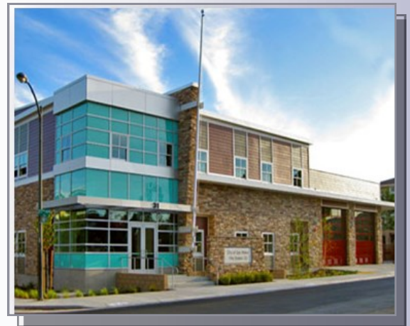
San Mateo Station 23—31 West 27th Ave. Engine 23—3 personnel; Truck 23—4 personnel BC5
