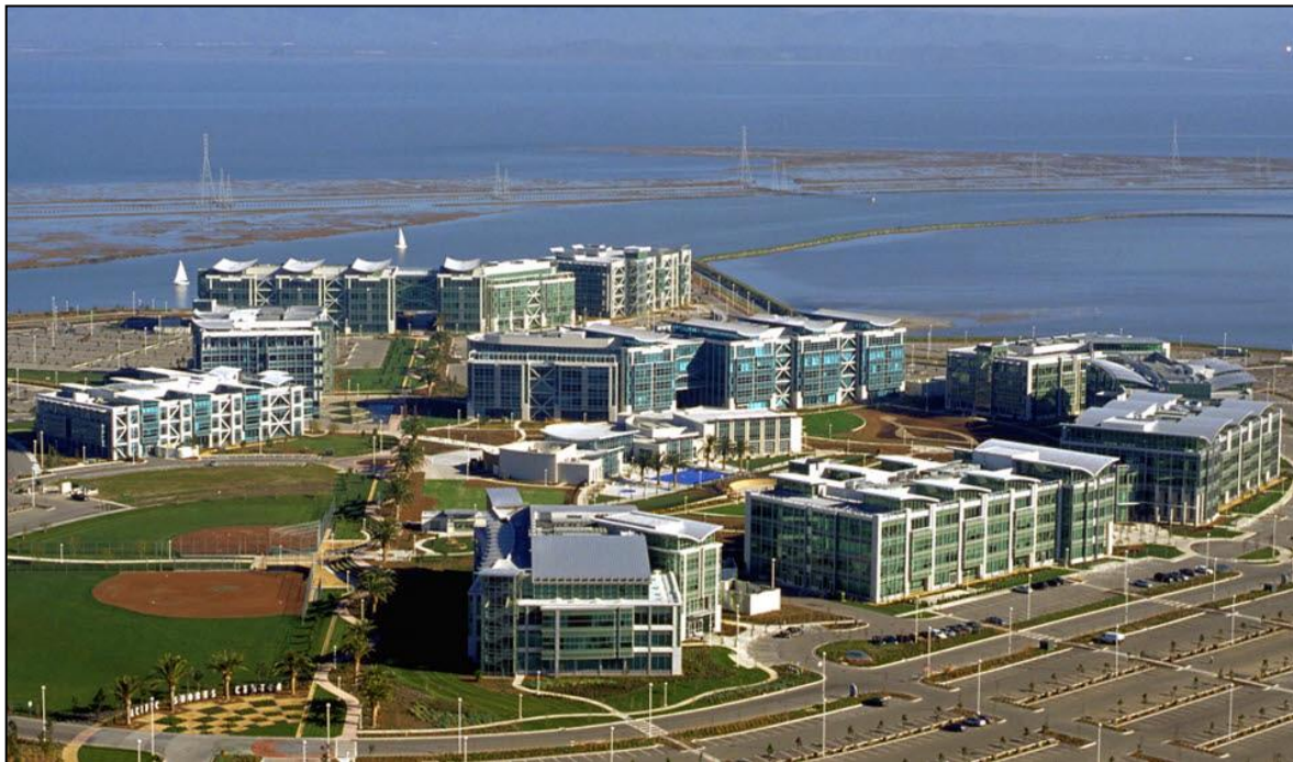
Fig 5.2 Example of building height hierarchies. Note the range in heights from the one story amenities building to the 5 story building office/R&D buildings.
