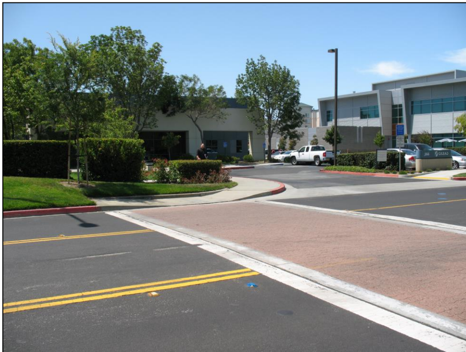
Fig 3.4c Example of clear demarcation – different paving materials –where walkway intersect with roadway
