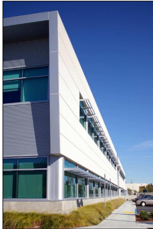
Fig 5.3a Building with contemporary identity: 362 Vintage Park Drive
