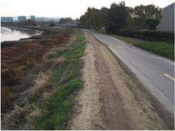
Segment 7 looking south towards Gateshead Park
