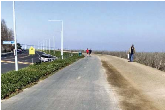
Earthen levee along Beach Park Boulevard
