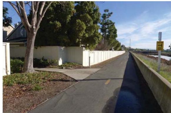
Raised earthen levee with concrete floodwall levee along the Bay Trail adjacent to Rock Harbor Lane
