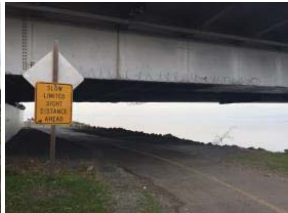
Segment 3, under the San Mateo Bridge/SR 92, looking northwest
