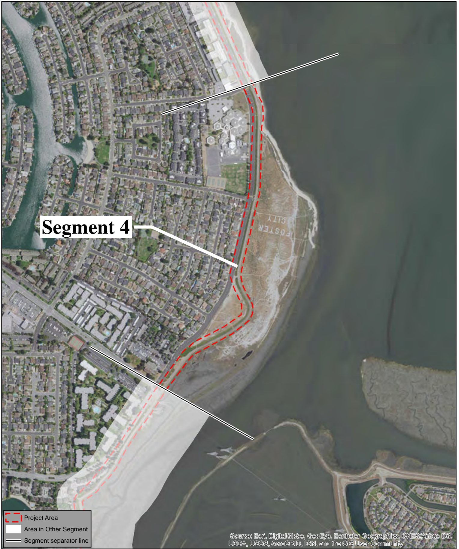
Figure 11d. Segment 4 Levee Overview
