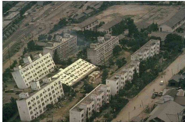
Liquefaction during the 1964 Niigata Earthquake
