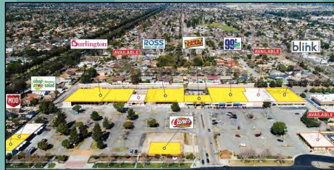
Upland Village – After Repositioning
